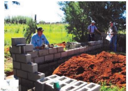
The team laid up the block walls, put the roof on, poured the floor, did the plumbing, put in a partition, and plastered the walls—all in 8 days!
